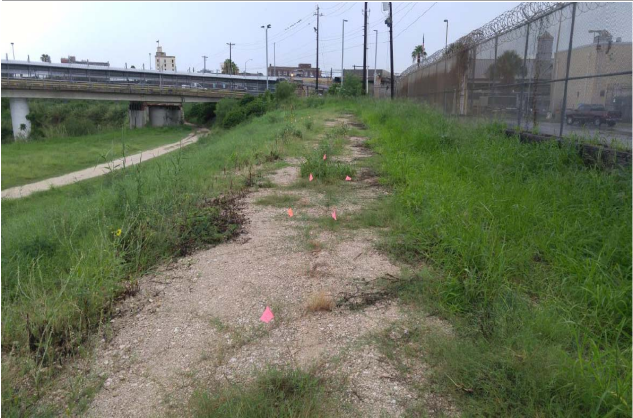
Photo 2 - Looking North - Surface Tension Crack of Pin Flags 5B through 10B.
